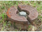
connects to the water supply. The water main entry valve to the aqueduct network which sticks out of the ground at the front of your property, commonly called "bottle" is buried underground, generally in front of the residence, usually at the the limit of the property between the municipal and the owner's properties. It is therefore very important that this entry valve be visible and accessible at all times. None other than a municipal employee is authorized to handle this water hook up.
